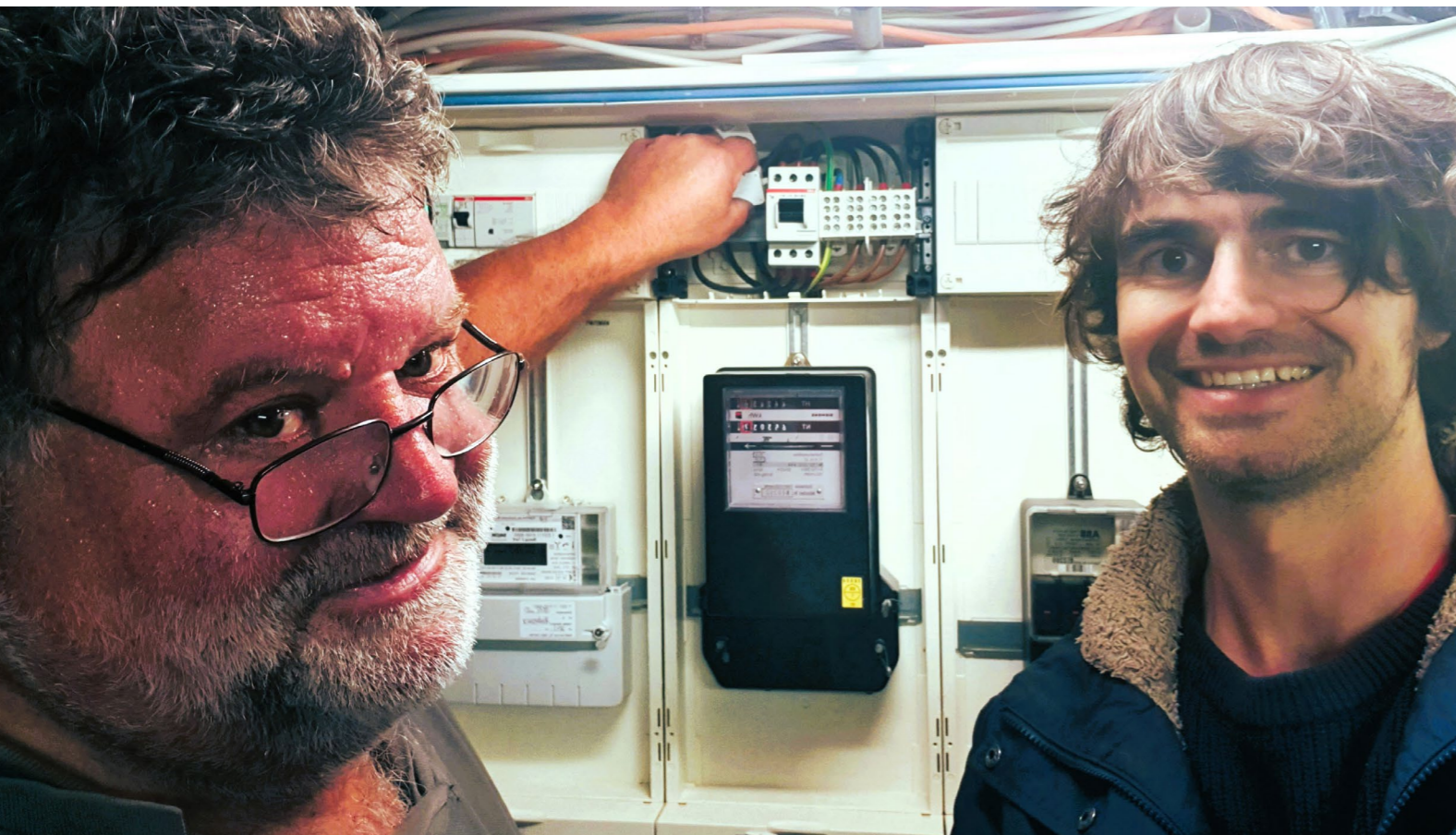
Figure 8. Installation of intelligent metering systems at citizen scientist household (Ph: WECF)
